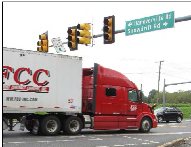
Vertical clearance for the signal heads at the intersection of Airport Road and Hanoverville Road is substandard, resulting in damaged signs and equipment
